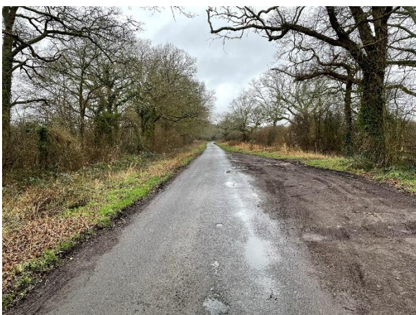
Graphic 3-1 View along Kent Street (Northbound)
